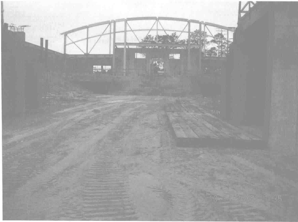
Figure I.5 The site work plan for this building was developed by CAD technicians.
