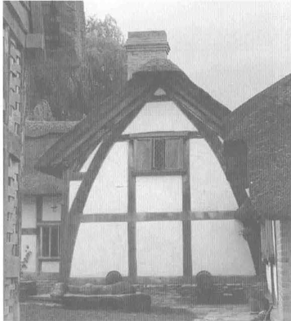
Figure 1.1: Photograph of typical cruck construction in Herefordshire.
