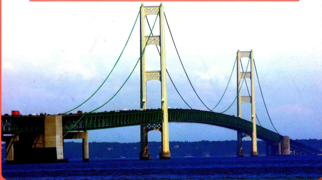
Mackinaw Bridge, Michigan © Ilene MacDonald/Alamy
