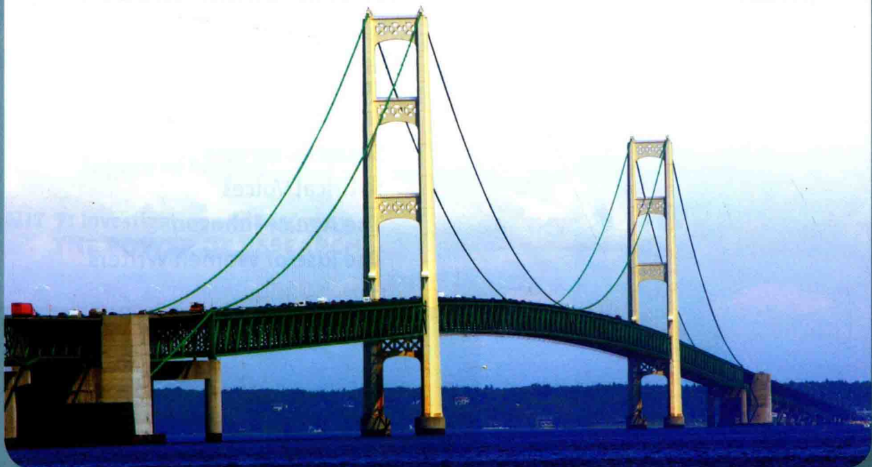
Mackinaw Bridge, Michigan © Ilene MacDonald/Alamy
