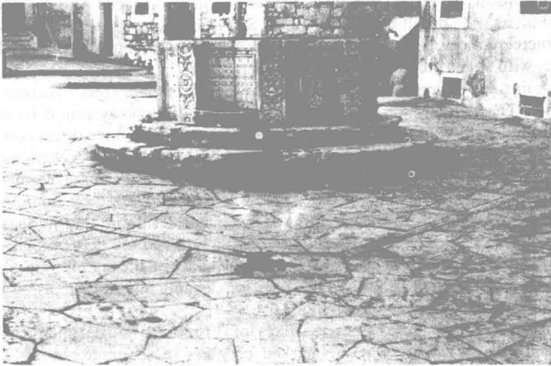
FIGURE 1-1 Venetian cistern head located at Dubrovnik, Yugoslavia, showing a stone grating.
