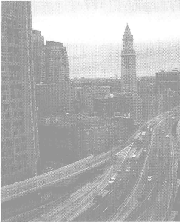
1.7 Highways of the urban renewal era often cut large swaths through dense older neighborhoods. Courtesy Boston Public Library, Prints Division
