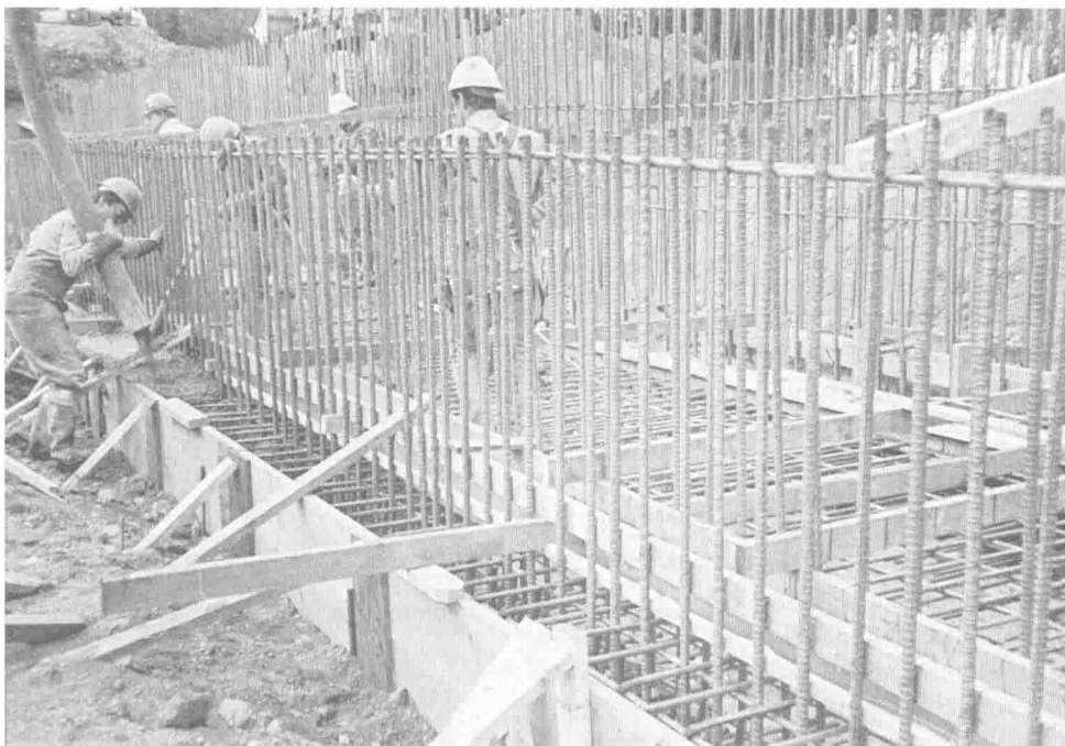
FIGURE 1-4 Concrete construction in progress. Note formwork, reinforcing bars, and pumping of concrete. (George Limbrunner)
