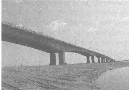
Fig.1 The appearance of the bridge
