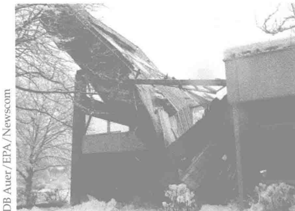
Figure 13 Failure from snow load.
