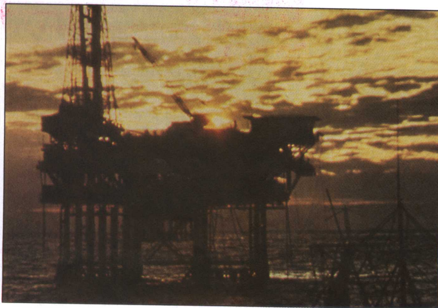
Offshore drilling platform. (Courtesy Sun Oil.)
