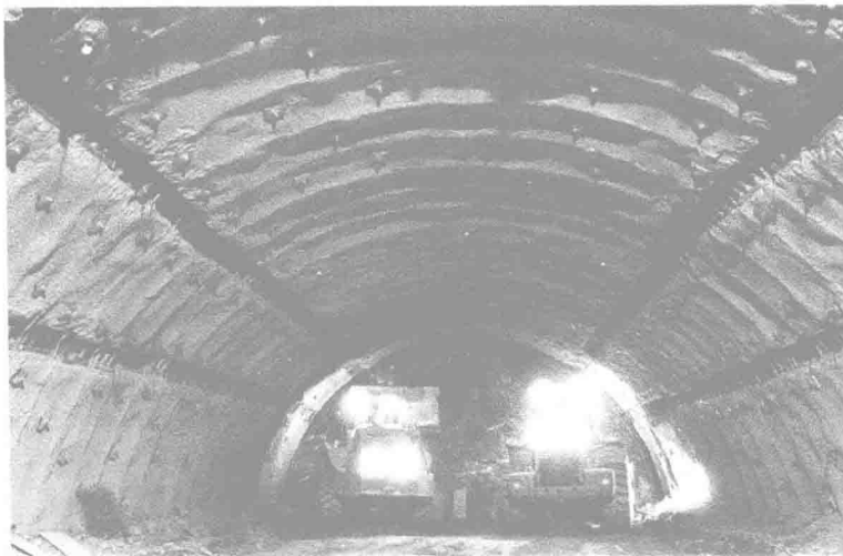
Figure 2 Yielding elements installed in longitudinal slots in the top heading [Photo: PORR Tunnelbau GmbH, Tauernntunnel, ASFINAG].
