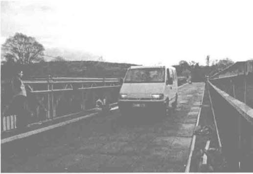
Fig. 3 Monitored bridge construction MABEY UNIVERSAL during the test
