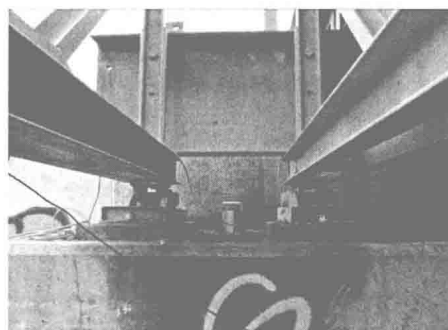
Fig. 2 Supporting of the structure on the reinforced concrete foundations
