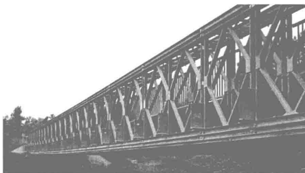
Fig. 1 Monitored bridge construction MABEY UNIVERSAL
