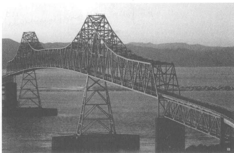
Fig. 1.4 This bridge truss consists of two-force members that may be in tension or in compression.
