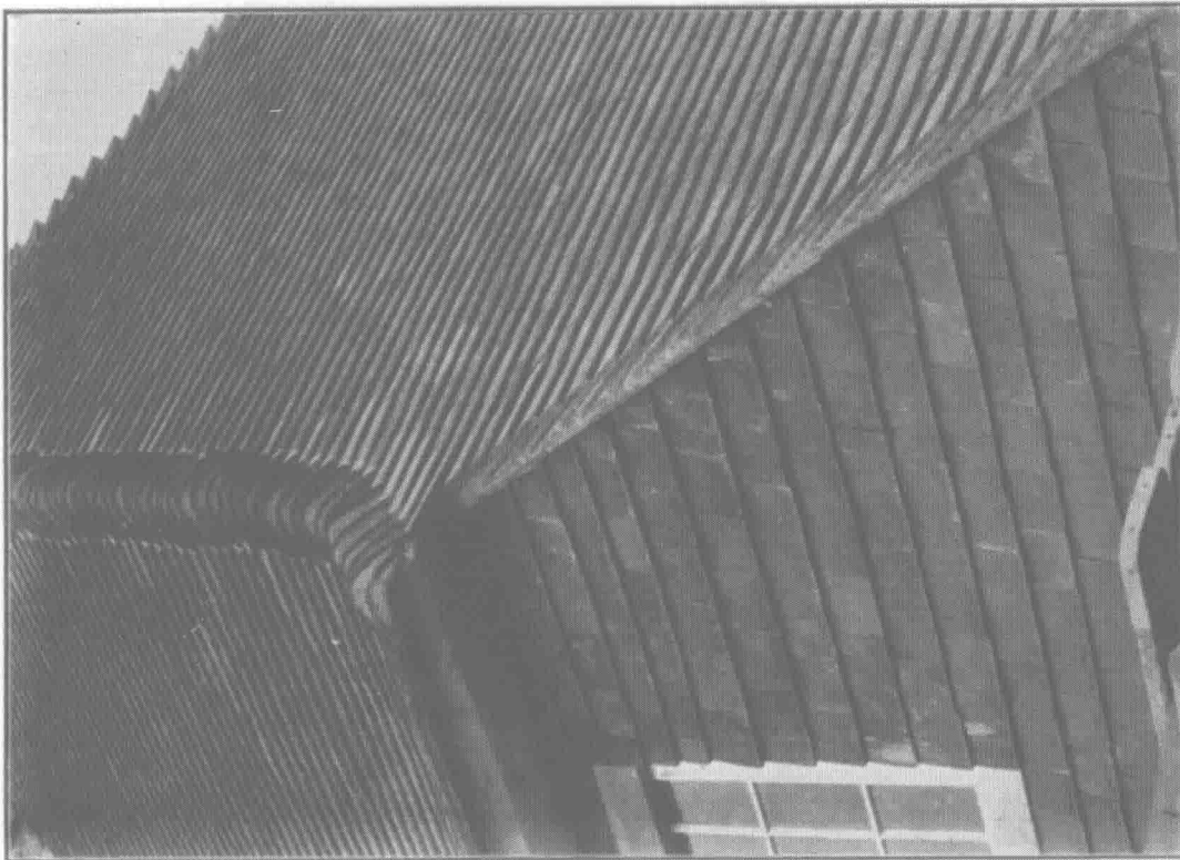
FIG. 12. (a) Right—and strong verge with undercloak tiles. (b) The board over the head of the window frame temporarily supports the heading course of wall tiles bedded in cement.
