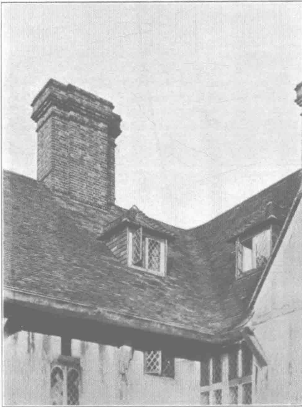
FIG. 20. Swept valley-tiles cut to wedge shapes.
