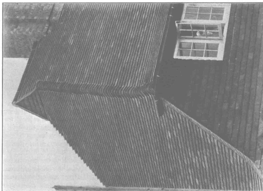
FIG. 3. Gablet, hip and verge treatments.
