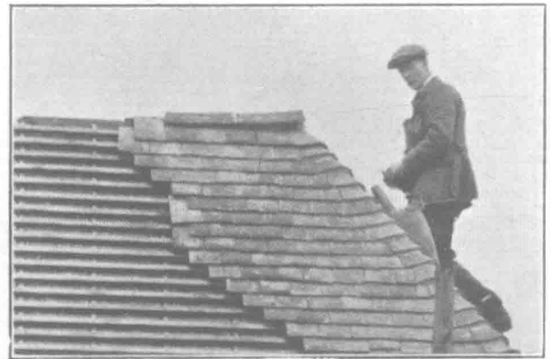
FIG. 21. Two faults are here illustrated. (1) The ridge tiles are not bedded down sufficiently closely. (2) The heading course of plain tiles and the hip tile of that course dip downwards instead of being tilted up slightly (as are those in the two courses below) to help the tilting of the end ridge tile.
