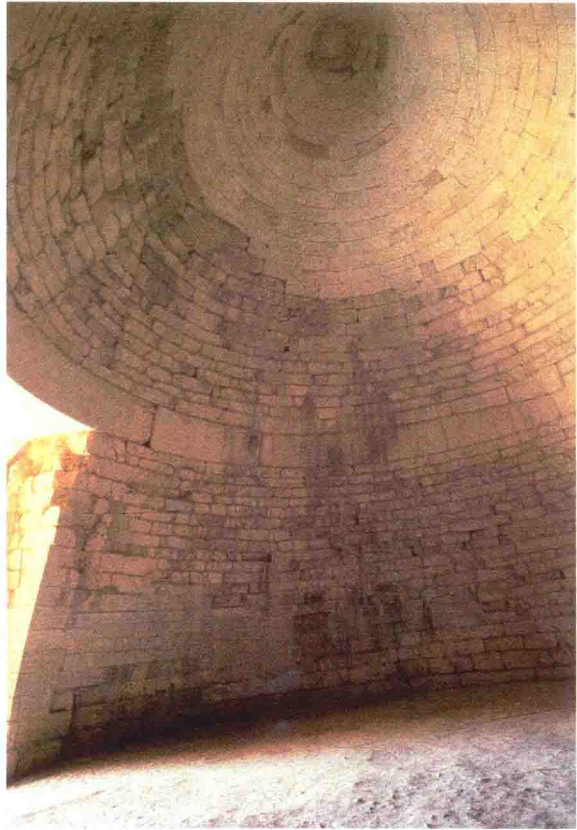
Fig. 1.5 View of the false vault in the Tomb of Atreus in Mykene, Greece
