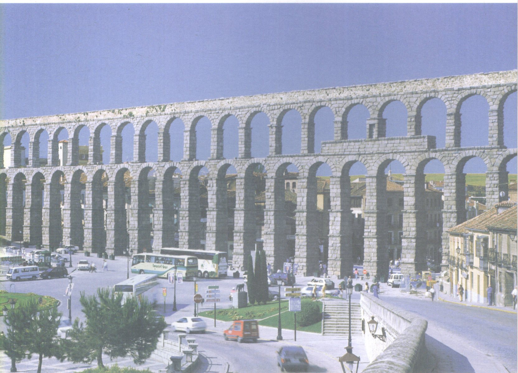
古罗马引水渠 Irrigation channel of ancient Rome
