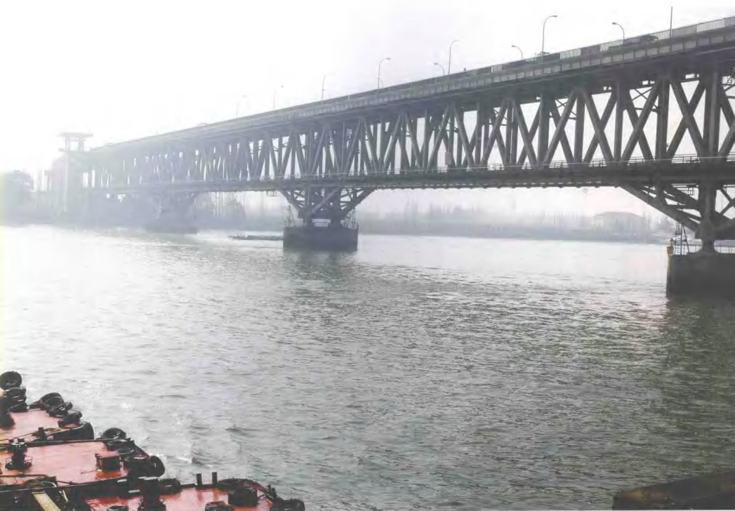
The First Bridge for Railway and Road over Huangpu River 黄浦江上首座铁路、公路桥——松浦大桥
