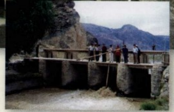
◎ 跃进引水渠首
