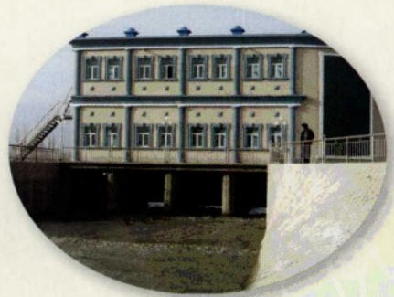
◎ 塔孜克电站分水闸房
