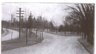
This road in Newton, Mass., is the heaviest travelled automobile route out of Boston. Nine years ago it was tarvated at a cost of 16¢ a yard, 1 mile, 16 feet wide, and is in fine condition today.
