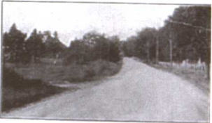
A section of this road at St. Joseph, Mich., was treated with oil and another section with Tarvia. After a year's wear the oil treated section has been worn down 2 inches below the Tarvia. Tarvia adds years to the life of any main road, as this experience proves.
