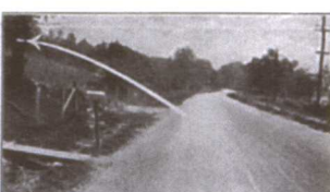
This Tarvia road at West Lafayette, Ind., was 10 feet under water in the floods of 1913, but that didn't hurt it a bit. The arrow shows highwater mark.
