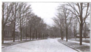
One of Cleveland's best residential streets (Belflower Road), tarvated with Tarvia in 1908. The photograph shows its condition in 1915 after 10 years' service without repairs.
