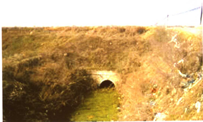
灌区污水集中排入排水渠
