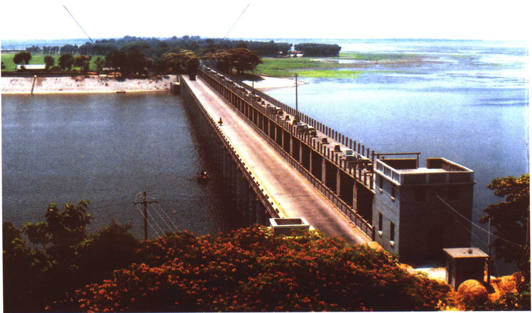
南四湖二级坝一闸
