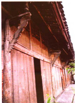
临街铺面 Street lining store facades
