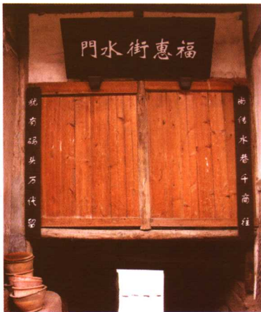
修复的水门 Repaired water city gate
