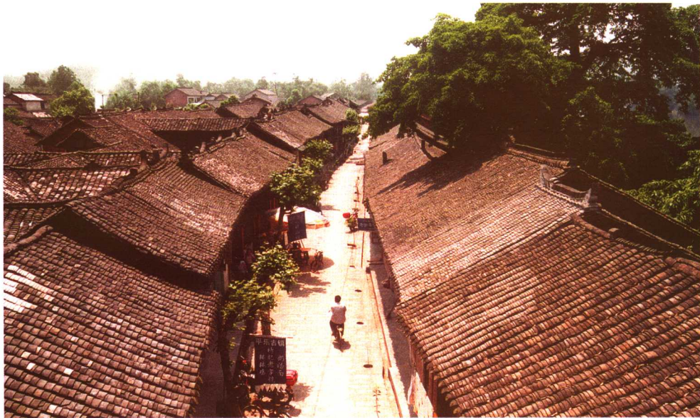
福惠街全貌 A panoramic view of Fuhui Street
