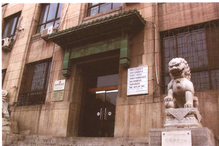
前门西河沿街交通银行旧址/Site of Communication Bank, Xiheyang of Qianmen
