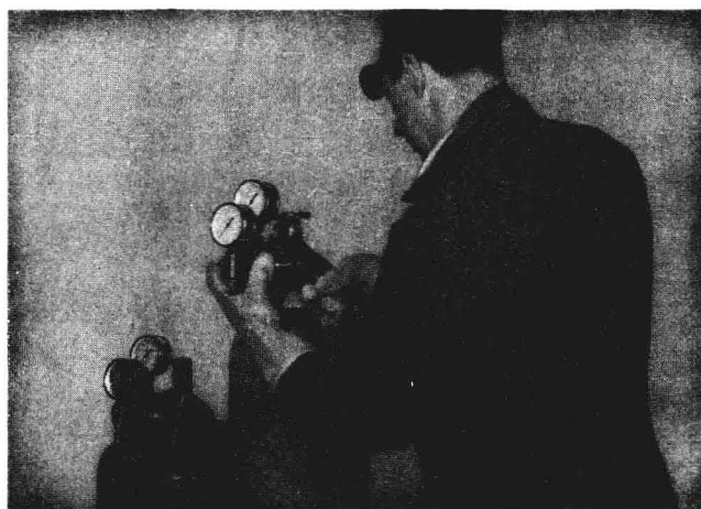
Fig. 7. Attaching the pressure regulators. To attach the regulators, connect the acetylene regulator to the acetylene cylinder and the oxygen regulator to the oxygen cylinder. Screw the nuts up tightly with a close-fitting wrench.
