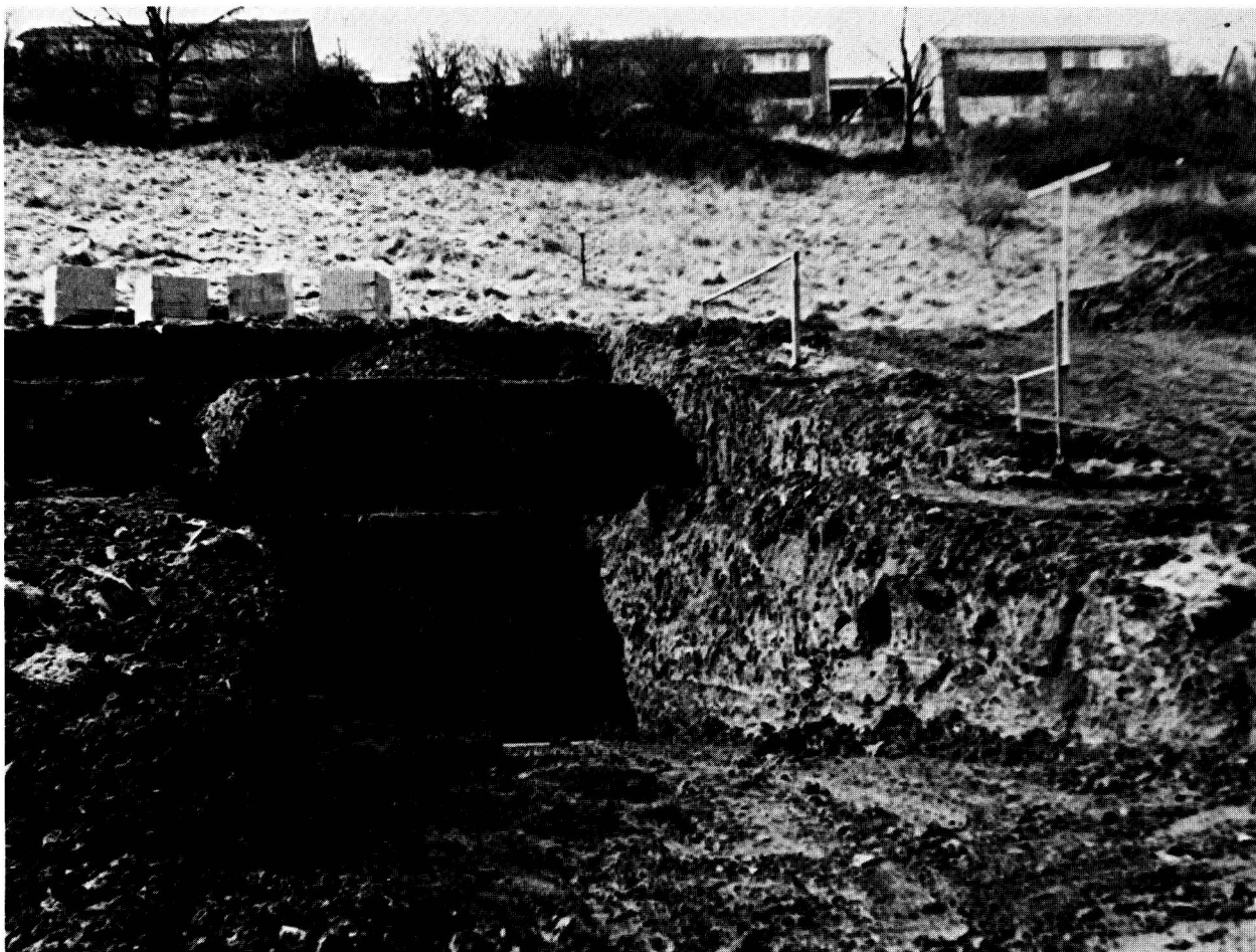
Fig 5. House foundations expose the underlying stratum and possible locations of clay.
