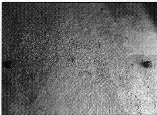
Photo 1.2 Not being controlled by the smooth mould surface, the inside is rough with a fibre pattern. Nevertheless it must be solid with plenty of resin, never fibrous, whiskery or full of pinholes. A glossy resin rich surface is even better. Note the nuts, not glassed over and accessible.
