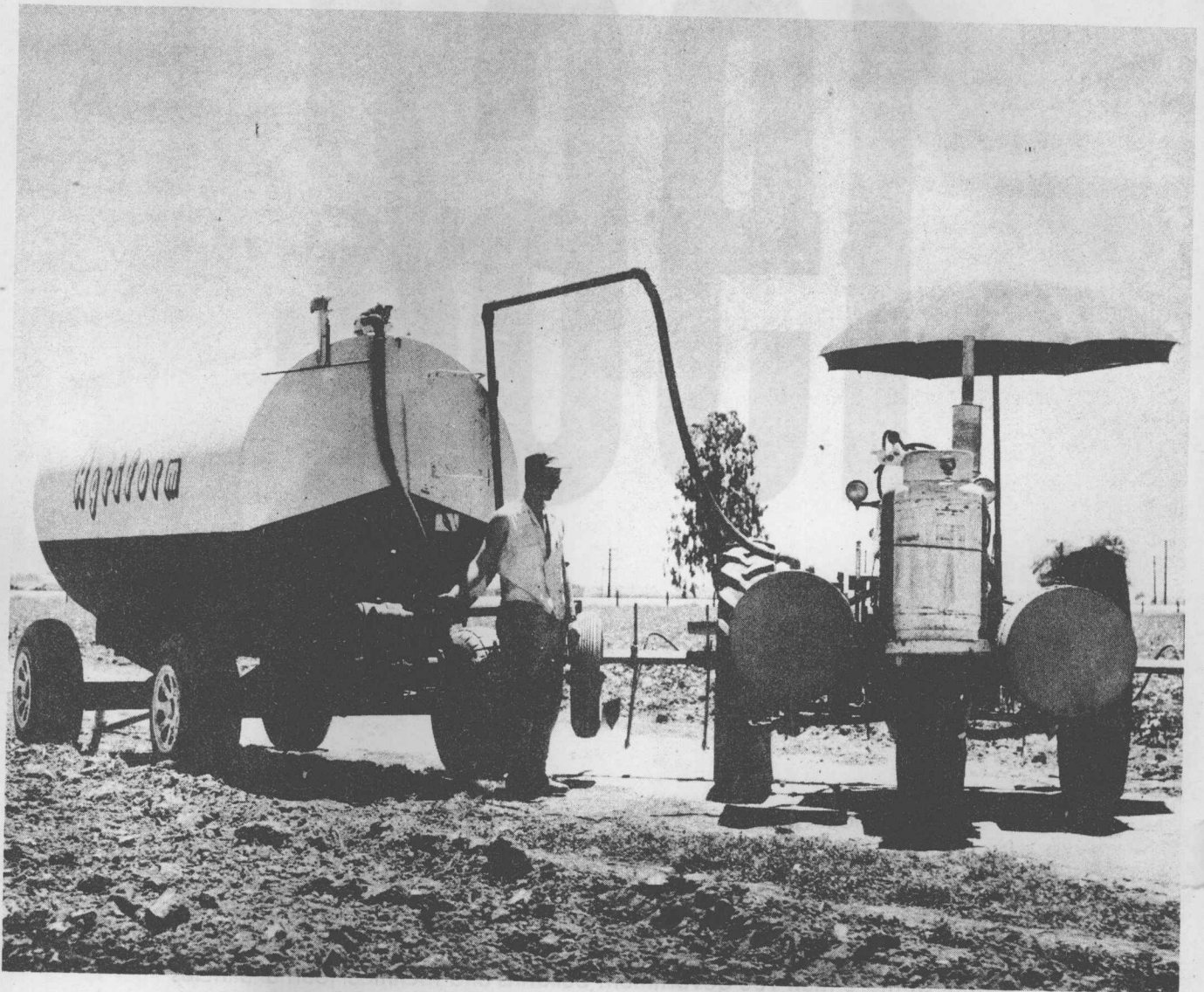
Custom applicator pumps liquid fertilizer from nurse tank to tractor-mounted applicator for use in cotton field.
