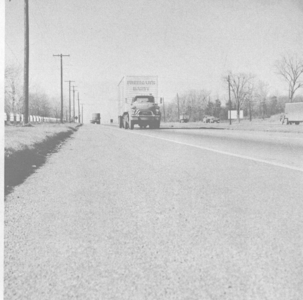
A soil-cement shoulder in New Jersey.
