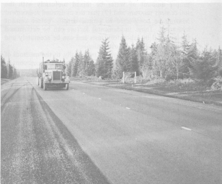
A soil-cement road in Washington.
