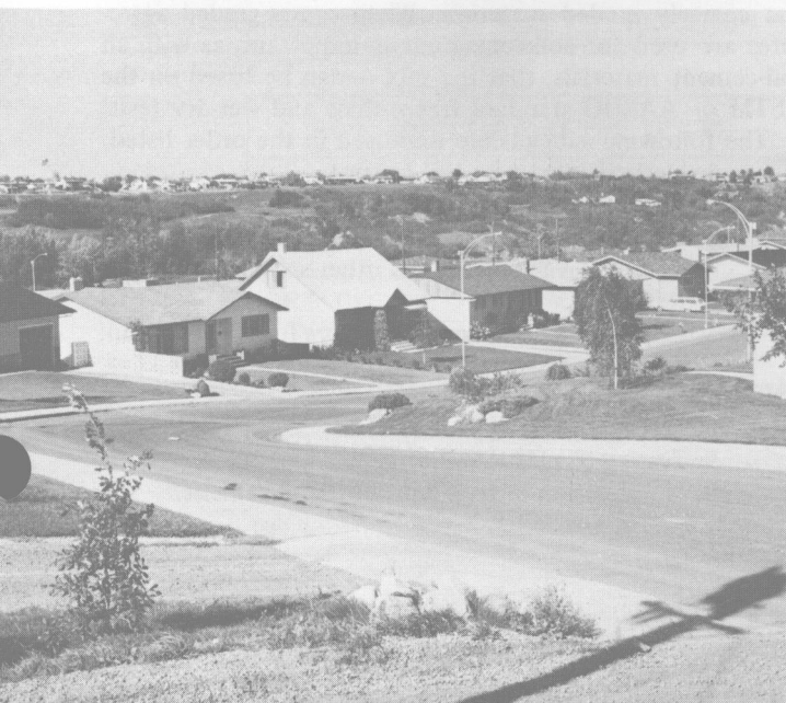
A soil-cement street in Edmonton, Alta.
