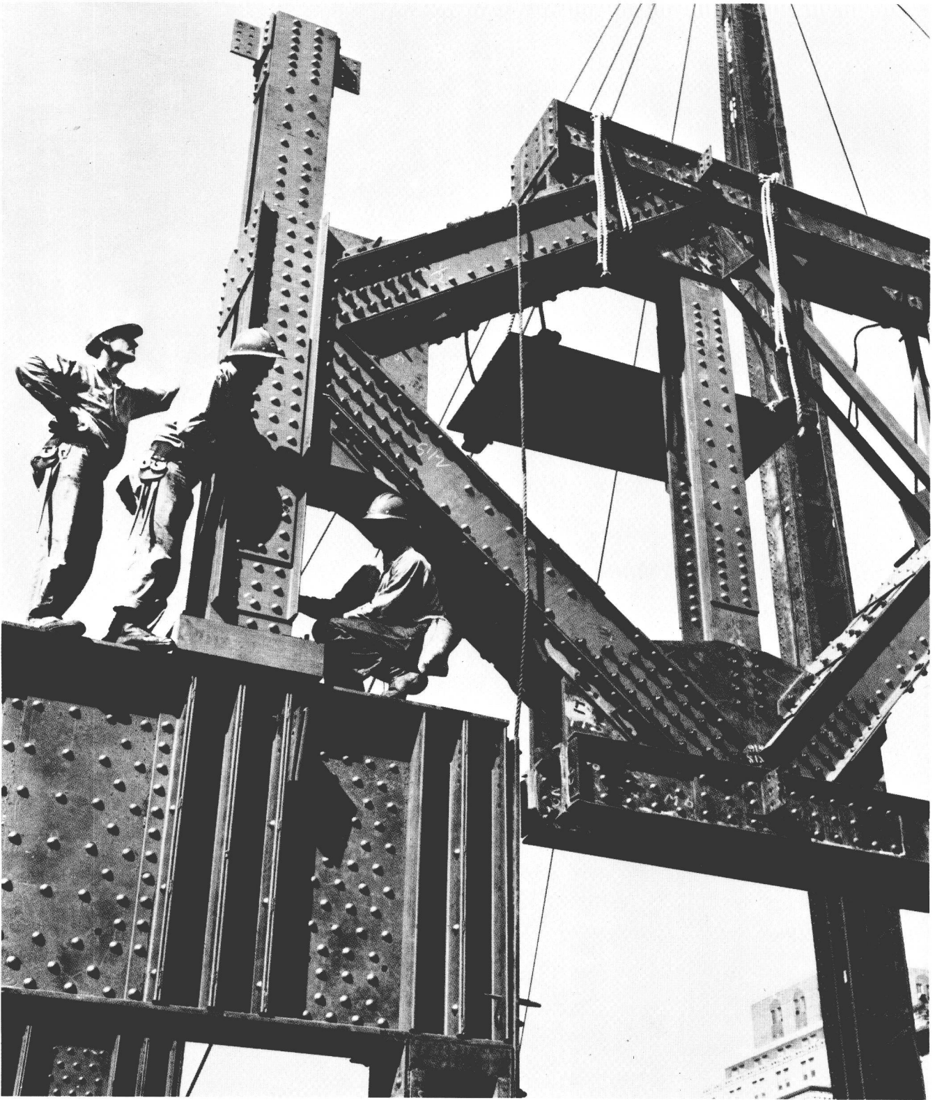
Typical industry photo. Hundreds of drawings were required to plan and build the hotel in which this 21.3 metre long truss was used. (Bethlehem Steel Corp.)
