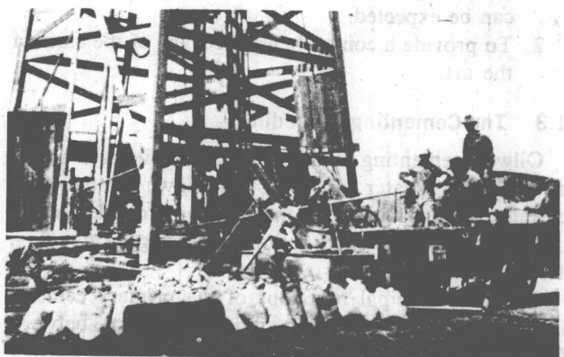
Fig. 1.3 Early-day cementing using sack cement.
