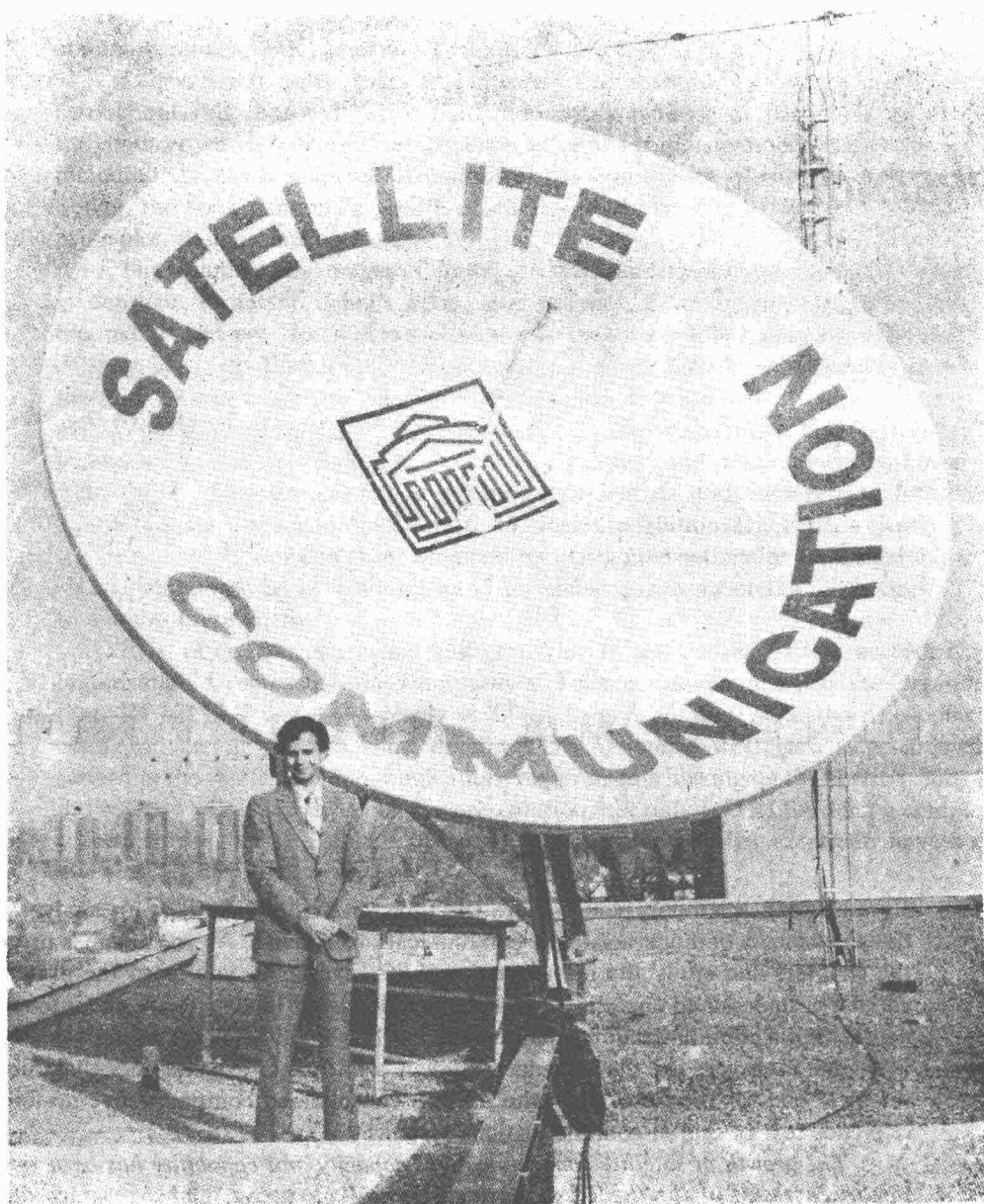
14/12-GHz transmit-receive antenna of the University of Ottawa. The performance of new modems, codecs and SCPC and TDMA systems is evaluated under the research direction of Dr. K. Feher. The Canadian ANIK satellites are used in these experiments. Professor Feher is in foreground.
