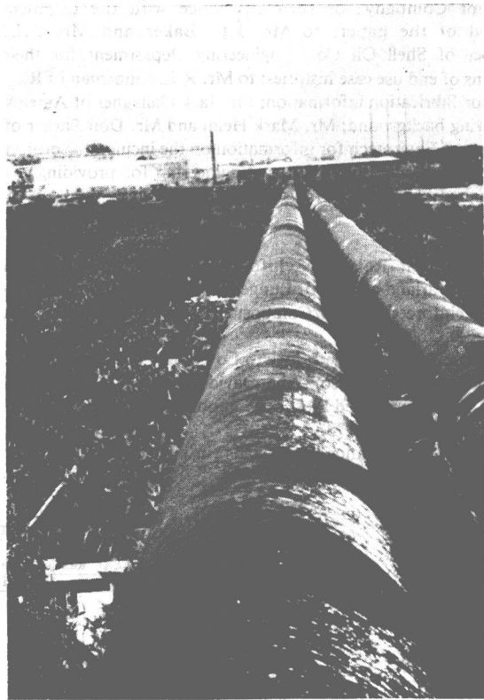
Fig. 2. Vinyl ester filament wound pipe 24'' and 36'' diameters
