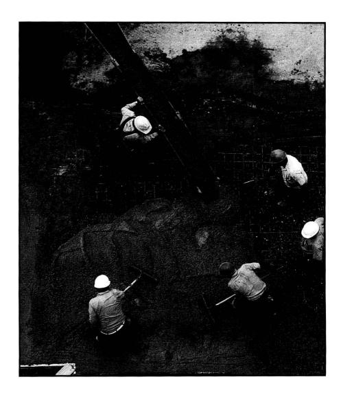
Sidewalks are constructed from separate concrete blocks rather than one continuous concrete slab, because concrete expands in the heat of the sun. Engineers must account for this expansion when planning the dimensions of the blocks.
