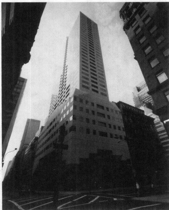
FIG. 2—This building is an example of conventional stone masonry on a concrete frame.
