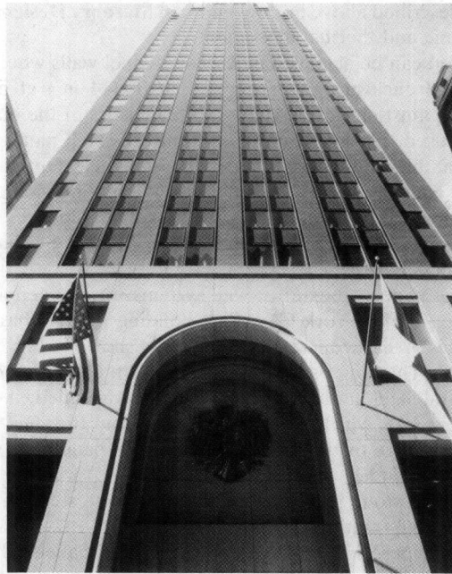
FIG. 4—This New York City bank building is an example of conventionally set masonry on a structural steel frame. The window system is a vertical strip design fit between masonry piers.
