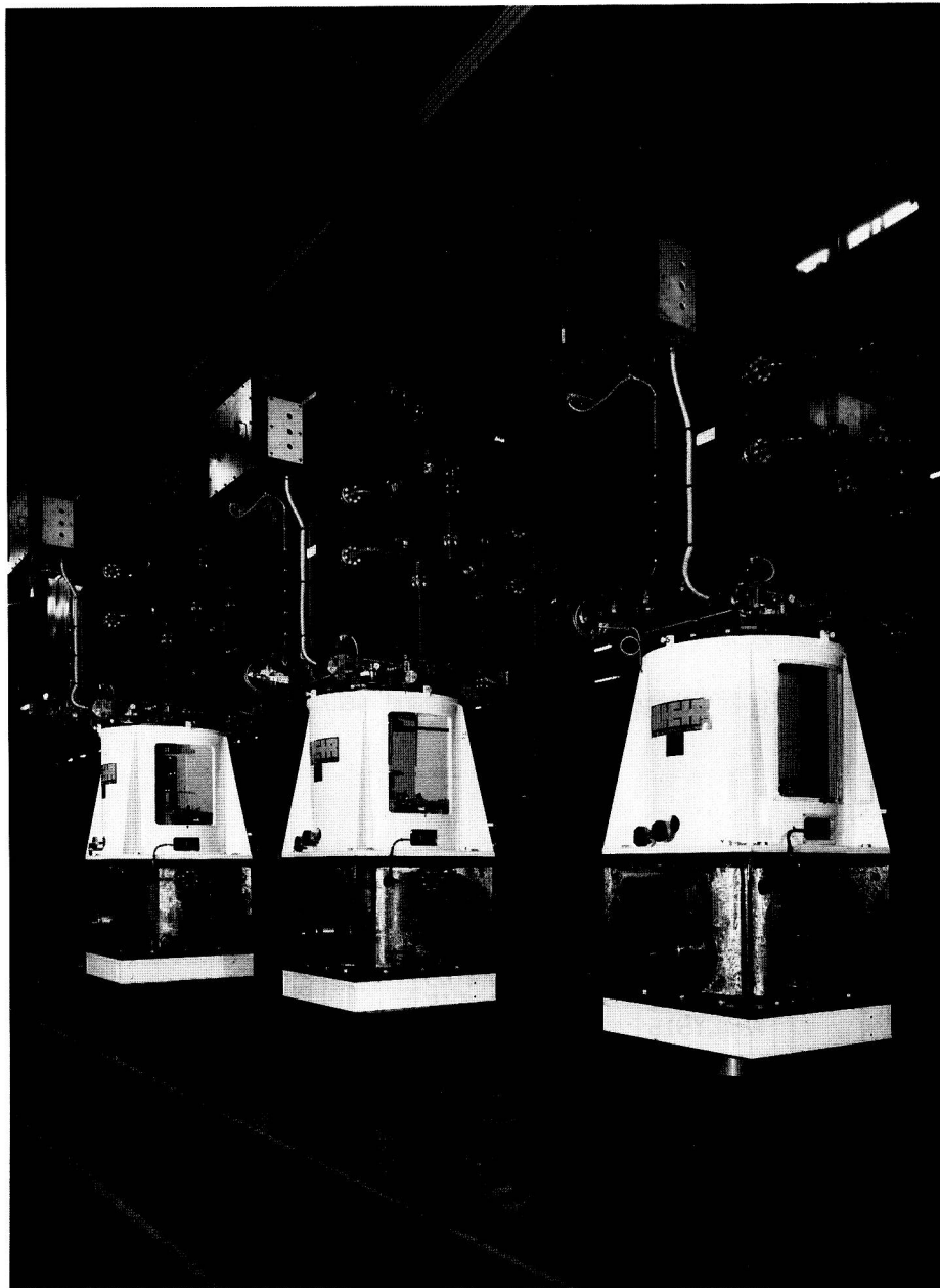
Fig 3 8"/10" Vertical oil export pumps 3.6MW at 3600 rpm
