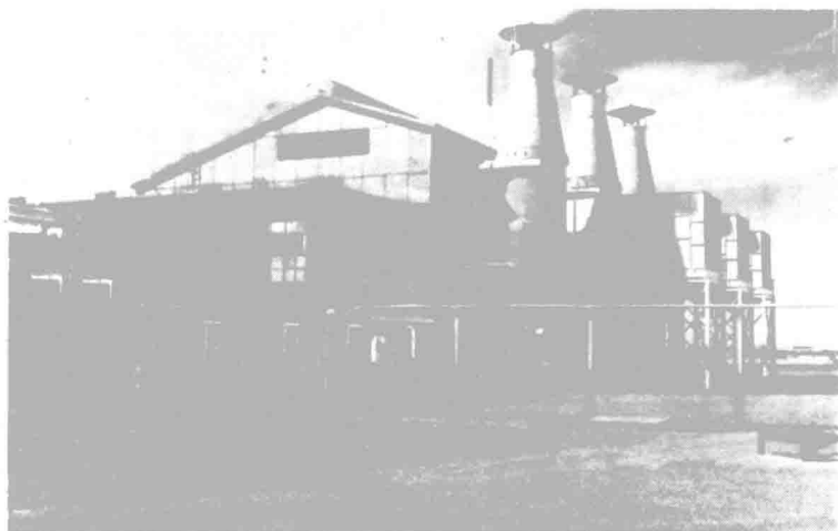
Fig. 1. Typical gas turbine station has three machines installed for series operation. Turbines are two-shaft, regenerative cycle driving centrifugal compressors and were designed for future automation.
