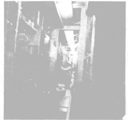
Fig. 6. Electricians and instrument men revamping existing panels.
