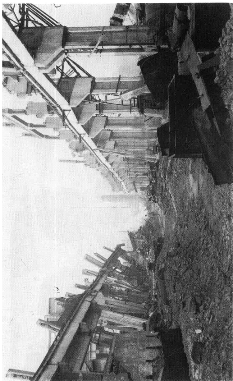
Damage to the steam locomotive engine factory by the 1976 Tangshan earthquake of magnitude 7.8 (photo by Rikitake, 1981).
