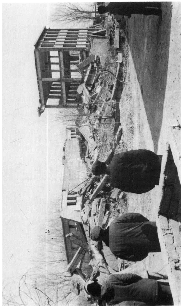
Damage to the library building of the Tangshan Mining College by the 1976 Tangshan earthquake of magnitude 7.8 (photo by Rikitake, 1981).
