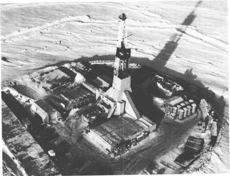
Fig. 1-4 Rig drilling on gravel island in Arctic waters.
