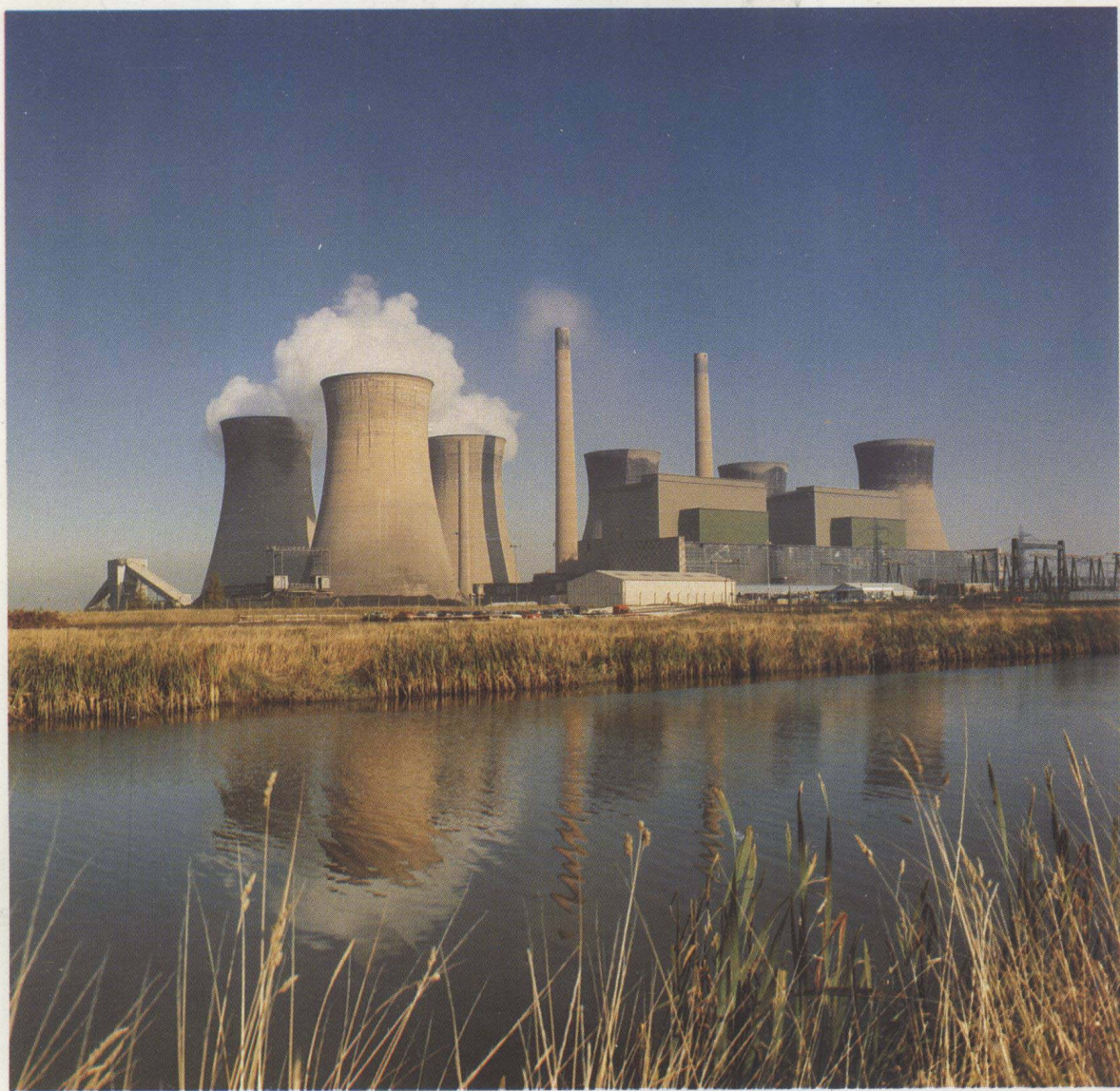
Natural draught water cooling towers at Thorpmarsh power station (simultaneous fluid flow, heat transfer, and mass transfer)
