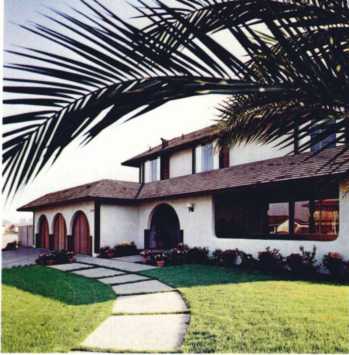
Fig. 1-12. Multimaterials and coordinated curves with straight lines give an architectural flair to this Spanish style home. (Brown and Kauffman, Inc.)
