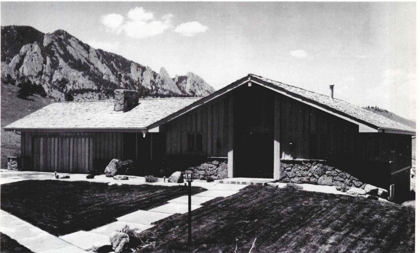
Fig. 1-21. Visible roof support is illustrated by the structural columns at the entranceway. (Marvin Windows)
