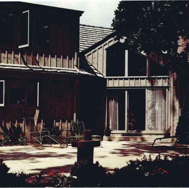
Fig. 1-16. The extensive use of wood for stained vertical siding and the split shake roof provide an attractive exterior for this home. (Marvin Windows)
