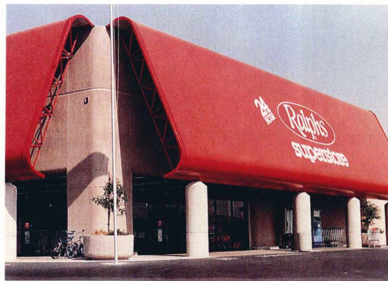
Fig. 1-2. Many commercial structures, such as this chain store, result from combined architectural design efforts. Note "Moduspan" slope roof with fabric cover. (Unistrut Space-Frame Systems)
