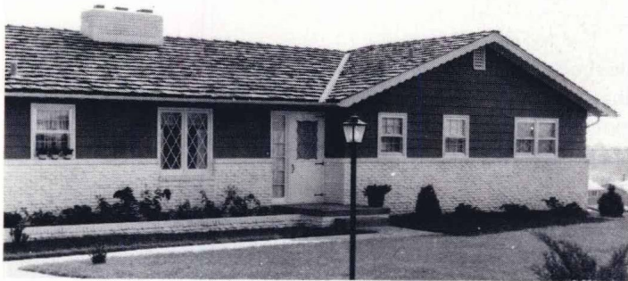
Fig. 1-13. A modern home with traditional characteristics including the overhanging gable, split shake roof, and grilled windows.
