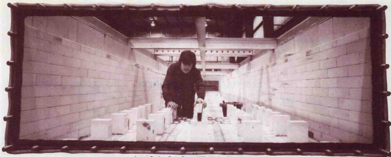
Large Pusher Type Tunnel Kiln Under Construction
