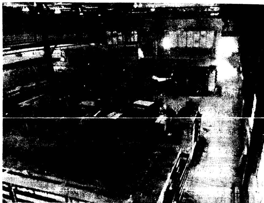
FIG. 6. Acheson graphitizing ovens: near oven under heat; center oven being packed; far oven being unpacked.
