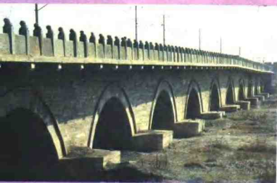
卢沟桥南面 The southern side of the Lugou Bridge
