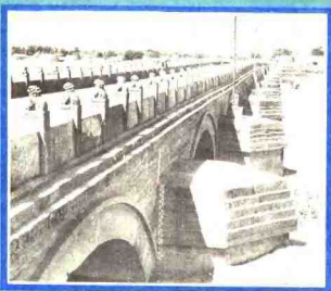
桥面及石狮、桥孔、分水尖 The northern side of the Lugou Bridge with its stone lions, arches and cutwaters.
