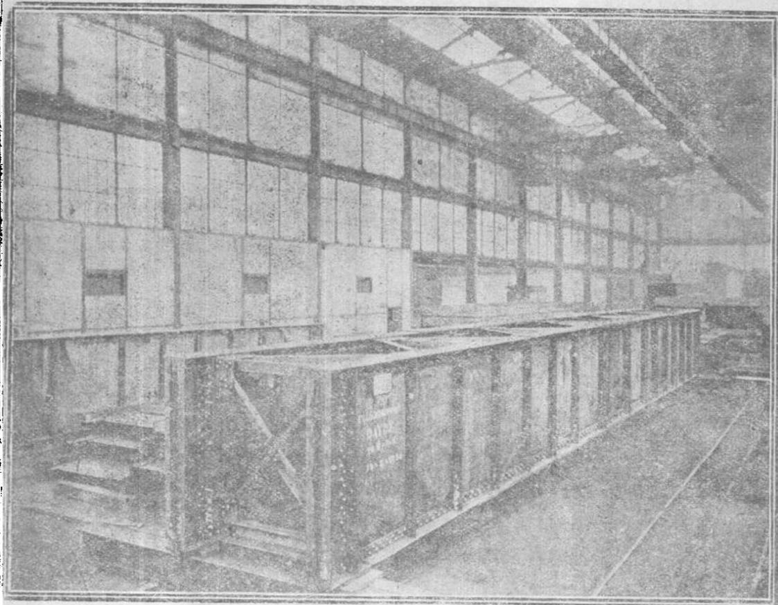
One of 20m. Steel Bridge Spans Supplied to the Ministry of Railways
