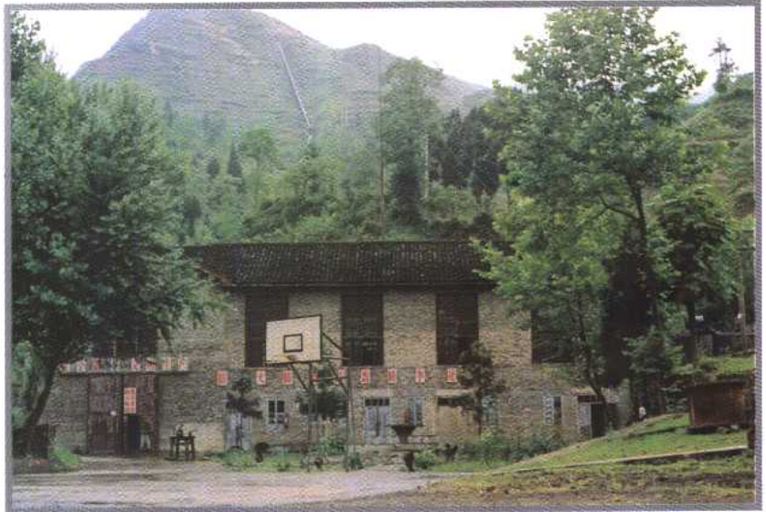
国营闹水岩水电厂
