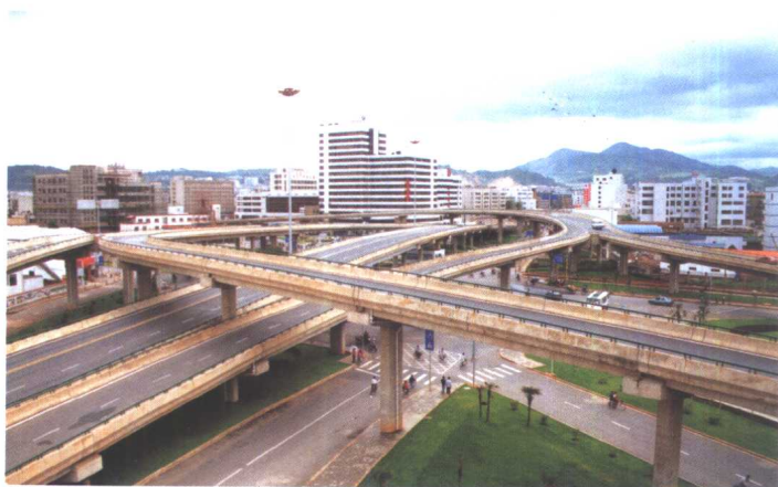
纵横交错的立交桥
