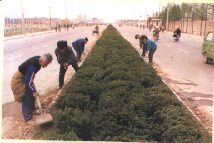
全綫開工修建中的楊高路工地 The construction site of Yanggao Road under its full line construction
