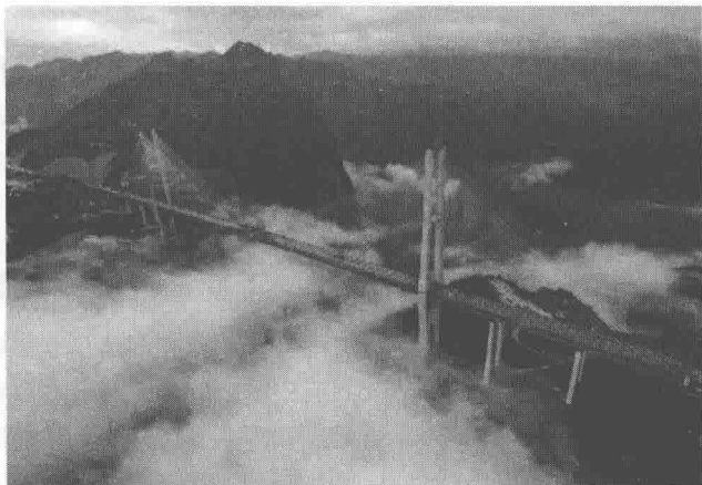
图2 杭瑞高速公路毕节至都格段的贵州北盘江特大桥 (来源: http://china.huanqiu.com/hot/2016-10/9516799.html )
