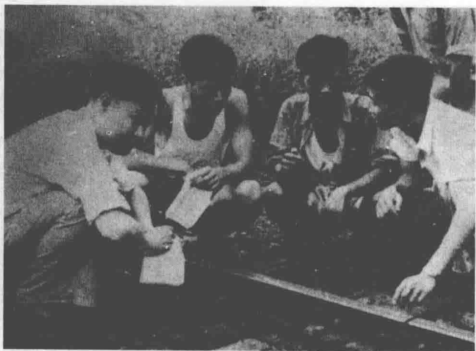
清华师生检查安装在石景山的球墨铸铁车轨
