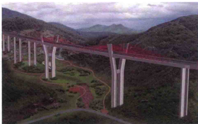
图 1.10 Pyung-Yeo 2 Bridge (平荣 2 桥)
