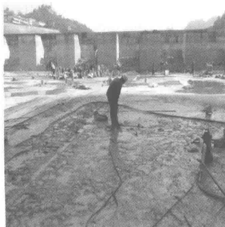
(c) 乌江沙沱水电站消力池
